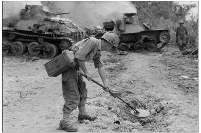
American sapper is looking for mines. Two Japanese light tanks Type 95 Ha-Go in the background
