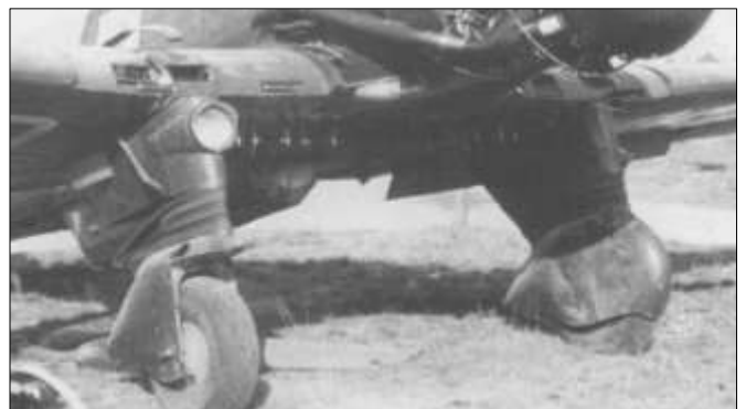
PZL 23 undercarriage detail
