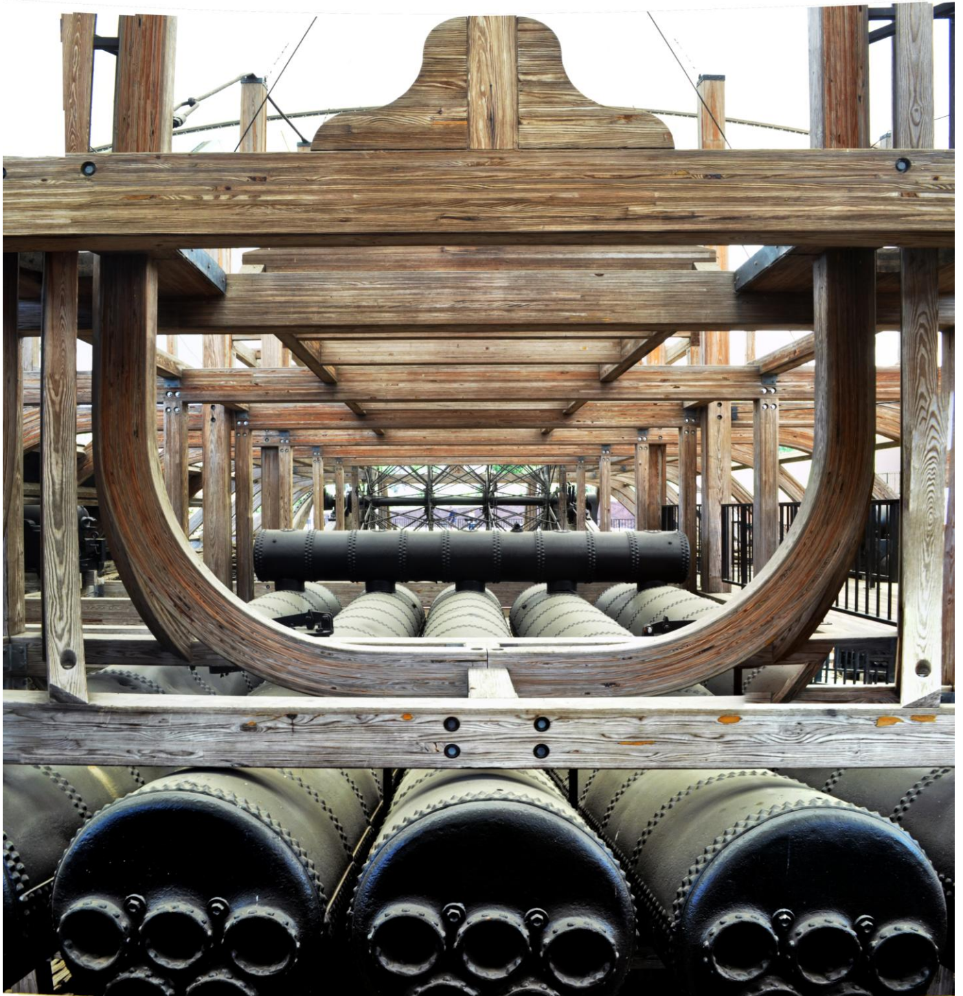
This three-shot composite photo shows the immense size of the boilers which are flanked on both sides by the pistons and huge connecting rods. In the distance, center, is the axle and steel arms of the paddle wheel.
