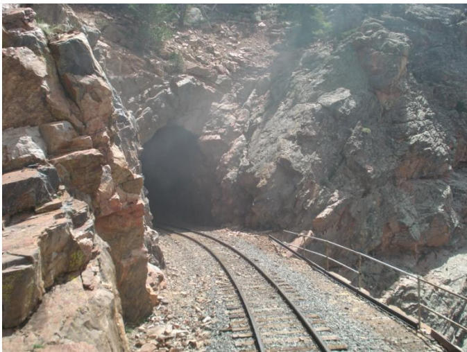
Exiting Rock Tunnel
